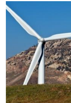
2.5MW Wind turbines
