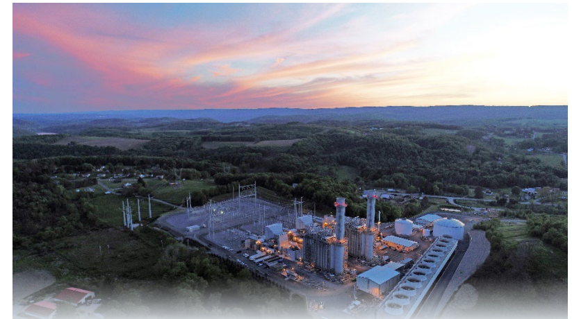
CPV Fairview Energy Center in Jackson Township, Pennsylvania using GE 7HA.02 gas turbines
